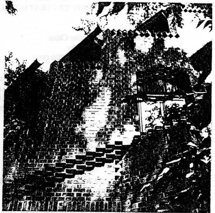
PHOTOGRAPH 2. BRICK CORBELING DETAILS
